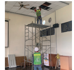
Photo of LED Lightening Installation at Rueifong Elementary School
