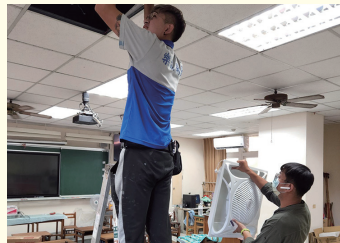
Unimicron and Love-Energy Industrial Cooperation in Construction
