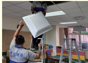
Unimicron and Love-Energy Industrial Cooperation in Construction
